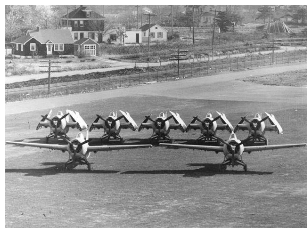
Fig. Grumman F4F Wildcat with STO Wing Folding Mechanism
